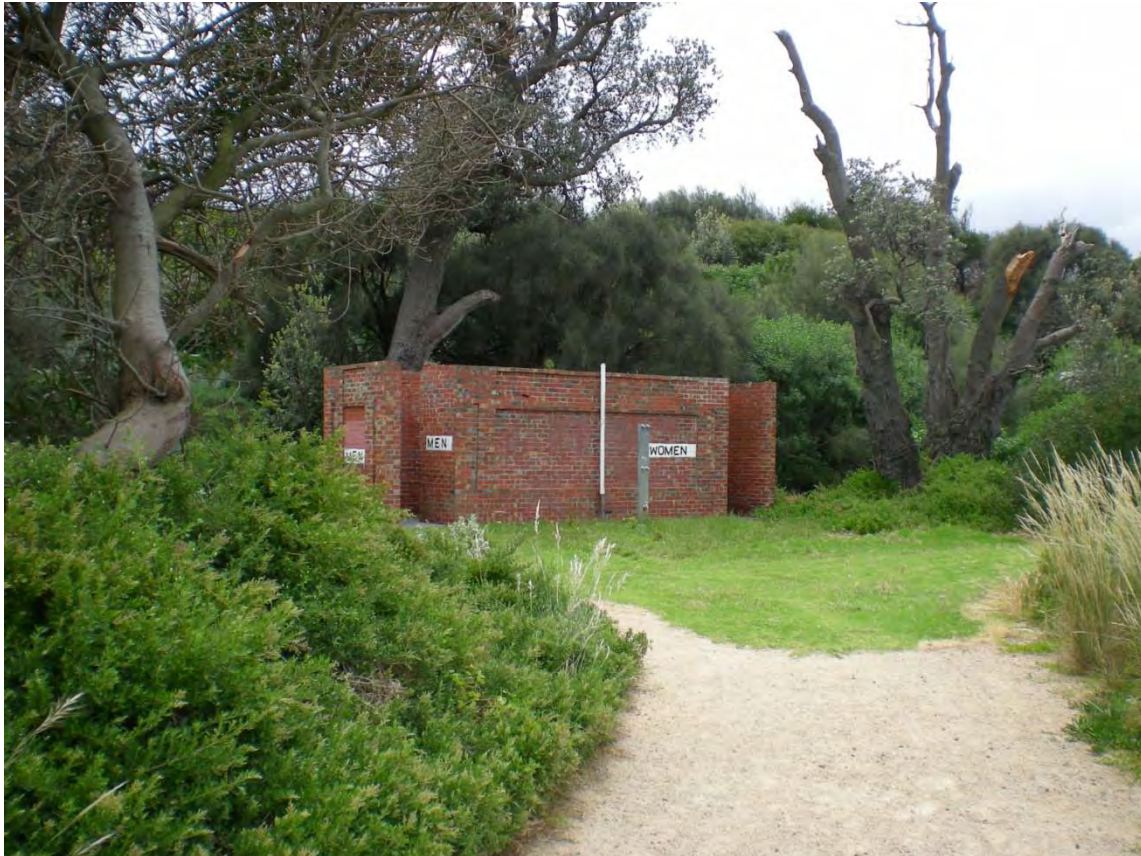
Figure 10: Beaumaris Foreshore Toilet (located near Beaumaris Life Saving Club)
