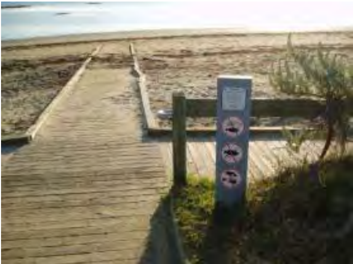
Figure 9: Disabled Divers Ramp
