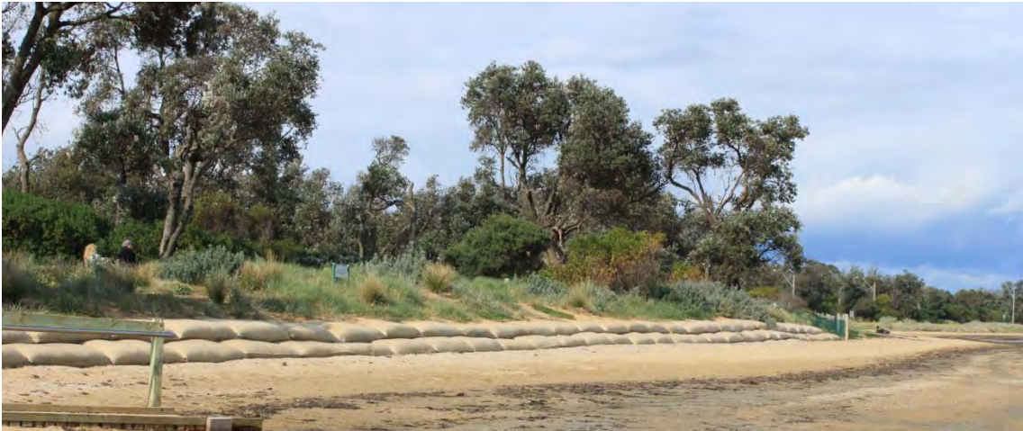
Figure 11: Sand dune stabilisation works, near disabled divers' ramp
