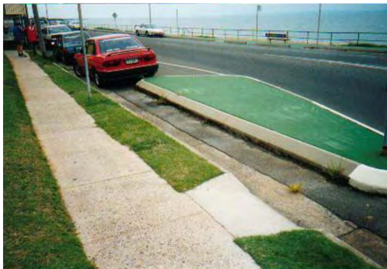
Figure 4.12: Parked vehicle blocks cycle bypass
