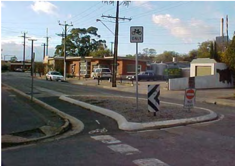
Figure 4.13: Cycle bypass at half road closure
