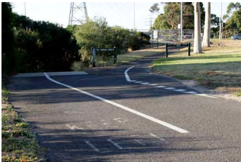
Figure E 2: The link path from Toorak Road joins at an acute angle, with restricted sight distance
