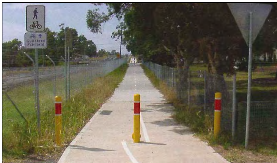
Figure 7.13: Example of a bollard treatment
