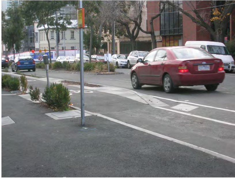
Figure 4.7: Kerb separated bicycle lane
